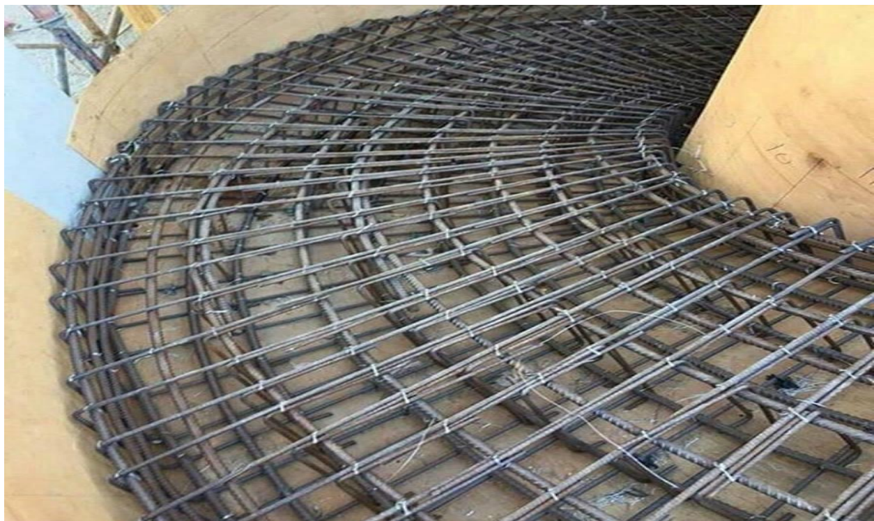
Fig 12 Curved stair concrete
