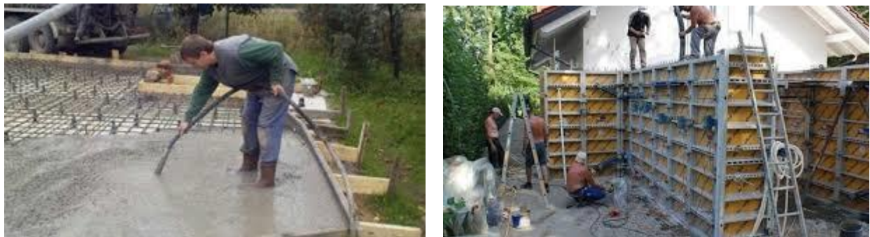
Fig 5 way of compaction
