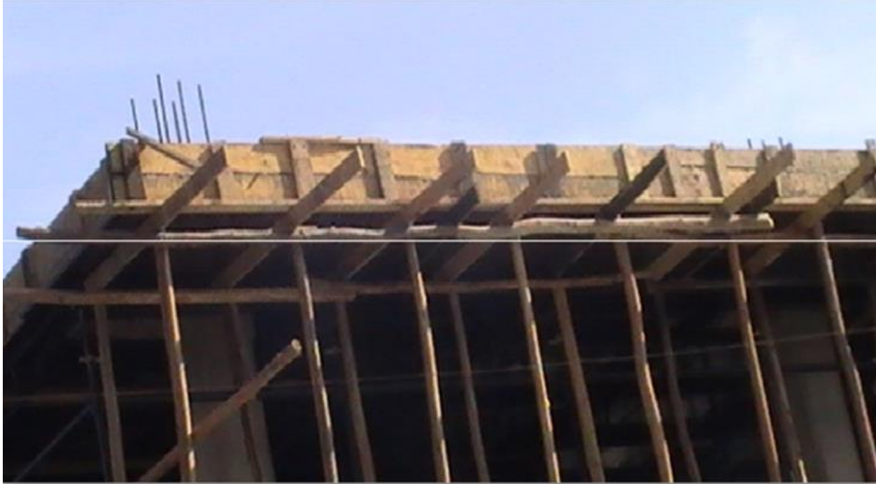
Beam and slab formwork
